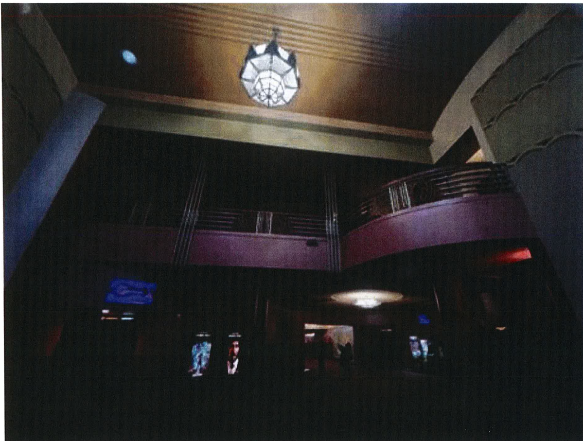
Mezzanine overlook, railing, and vertical elements.
